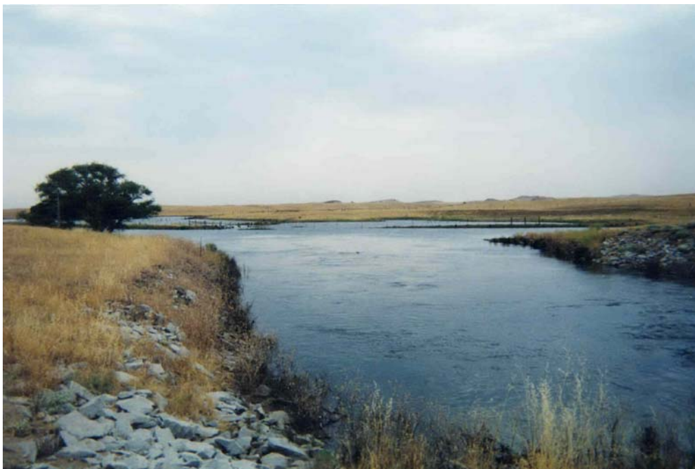
Photo 2-9. Start of the Madera Equalization Reservoir downstream of Hidden Dam
