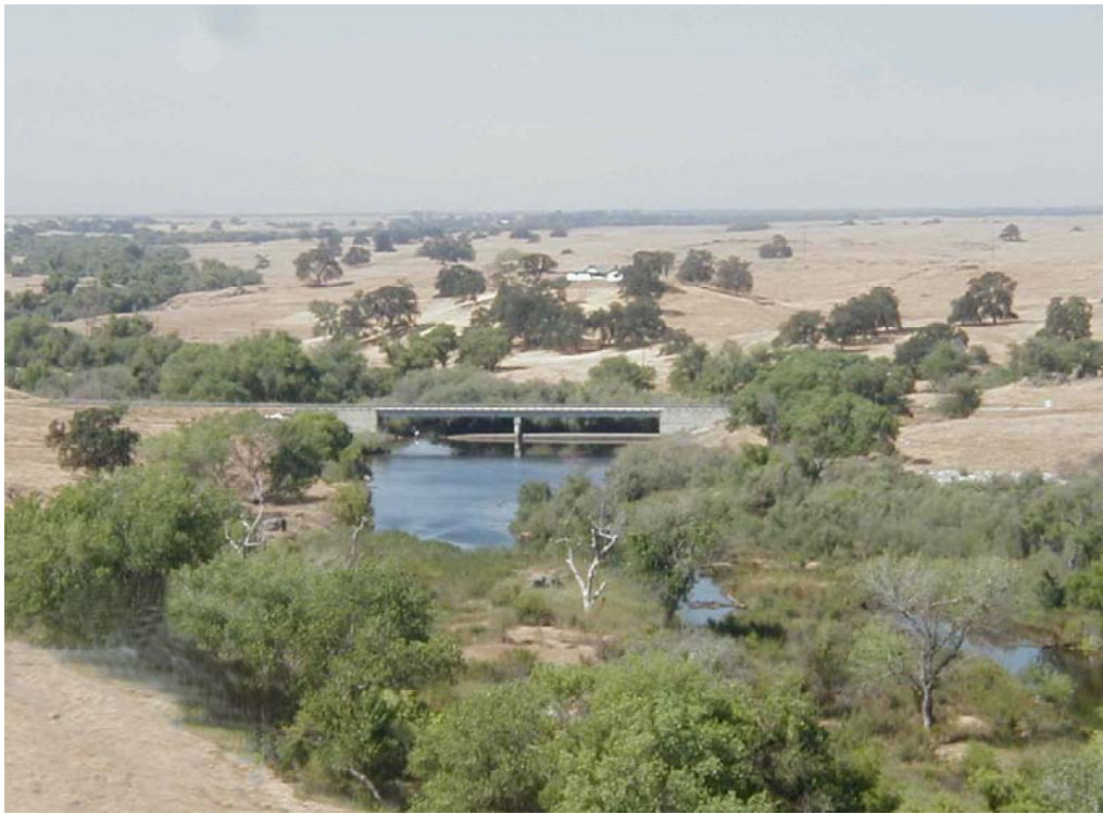
Photo 2-7. Bridge and weir Fresno River below Hidden Dam
