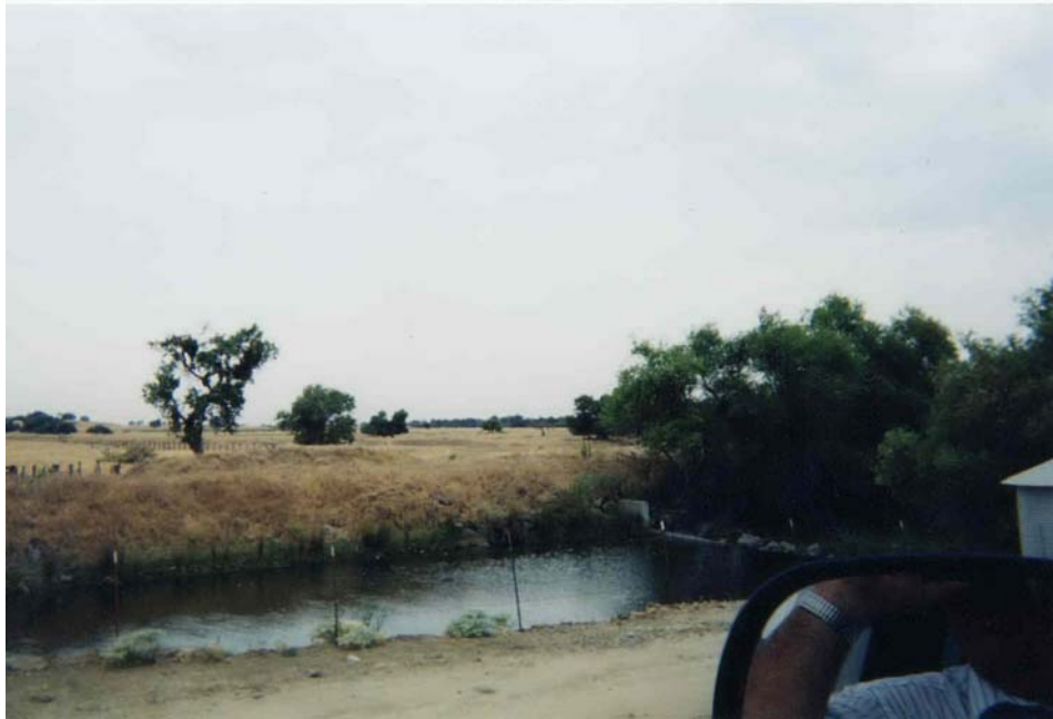
Photo 2-11. Cottonwood Creek levee at Fresno River
