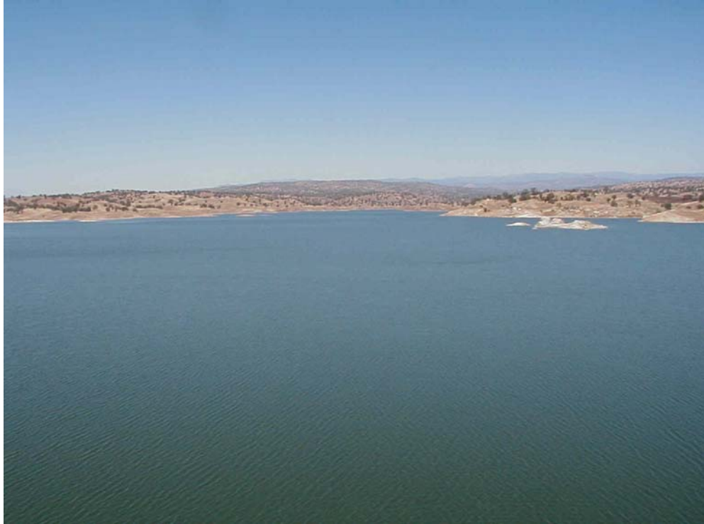
Photo 2-1. Hidden Dam-Hensley Lake looking north from the control tower
